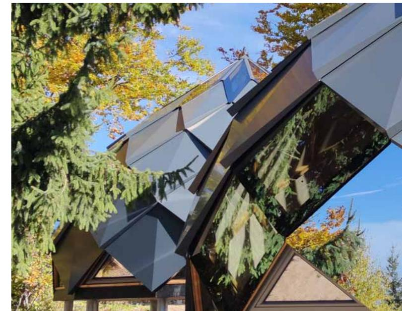
Each armadillo house is a raised on stilts above ground level with a timber diamond-shaped roof structure which extends from its top to the floor.
