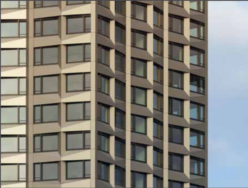
Depending on the light, the lustrous ALUCOBOND® PLUS anodized look C31 façade in warm, neutral tones changes colour subtly. | Picture: Florian Licht
