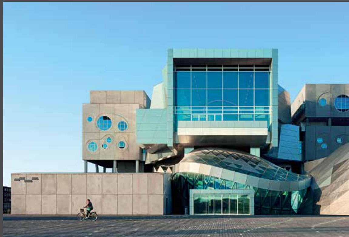
The ALUCOBOND® PLUS composite panel façade in naturAL Brushed gives the building its distinctive character. | Pictures: Duccio Malagamba
