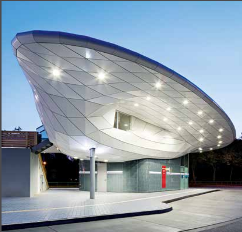
Poppenbüttel Bus Station's floating wing-shaped roof, made of ALUCOBOND® PLUS pure white. | Picture: archimages
