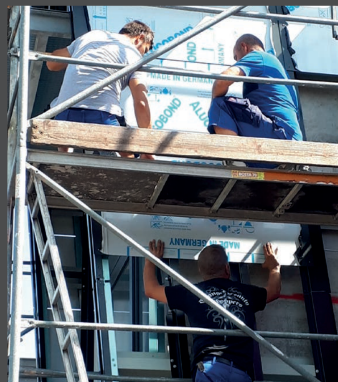
Easy installation of the ALUCOBOND® panels. | Einfache Installation der ALUCOBOND®-Platten.
