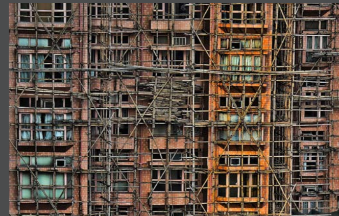
Bamboo Scaffolding | Bambuserüst Picture: Ricardo Gomez Angel
