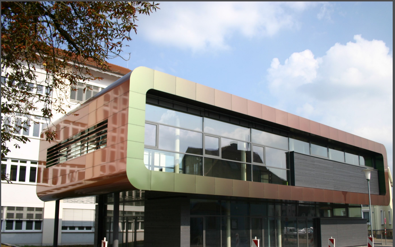
The modern extension stands out with its round forms. Der moderne Anbau besticht durch seine runde Form.
