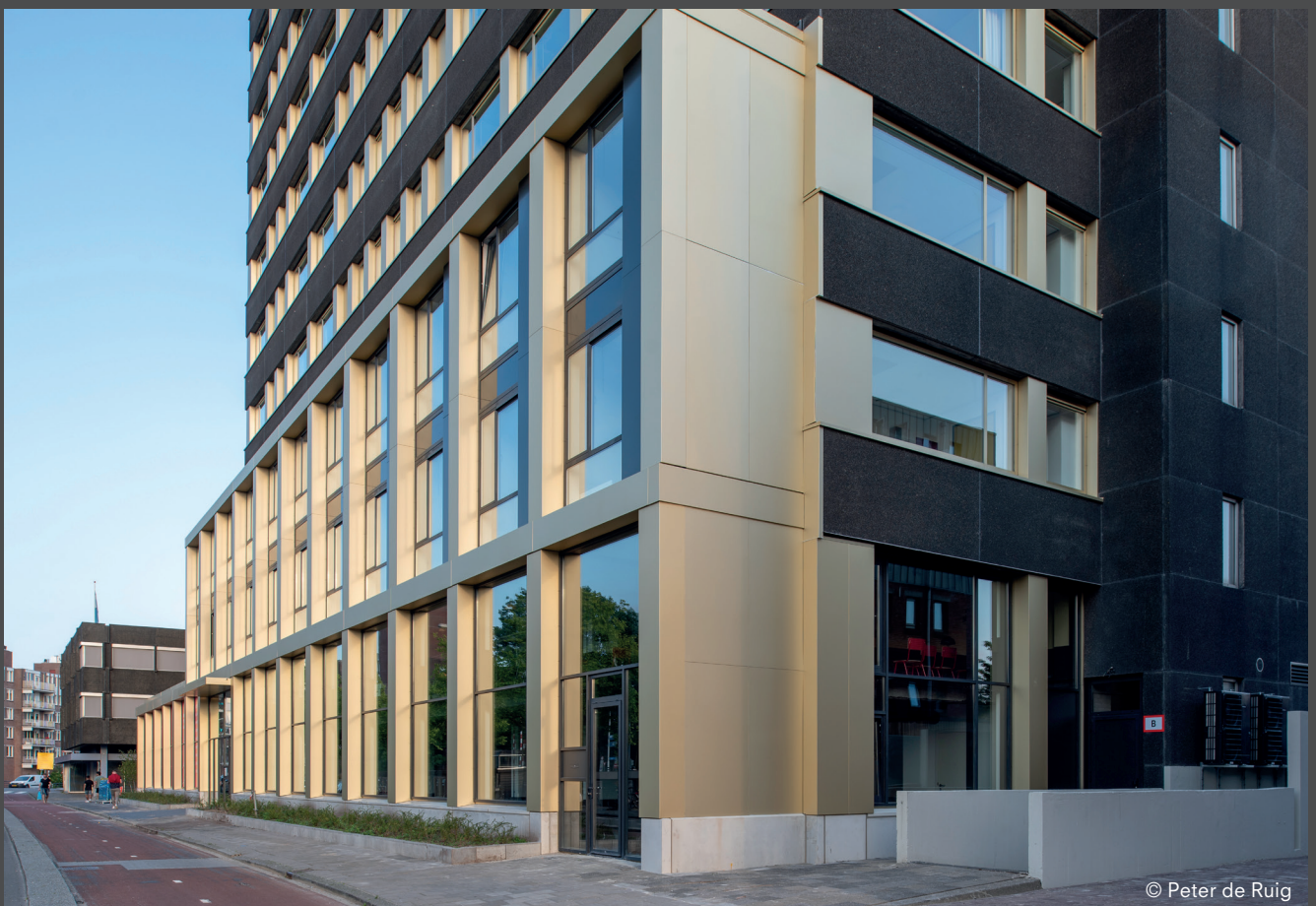
Black Box, Groningen | Team 4 Architects | Façade elements in premium anodised matt radiate supreme elegance.
